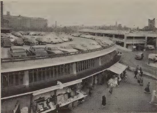
222 Coventry. The system of roof-top parking. There is interconnection from building to building.
